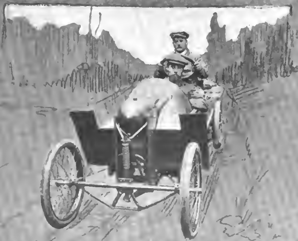
Front View Showing Motor
